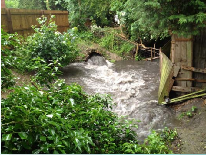
Culvert running full bore
